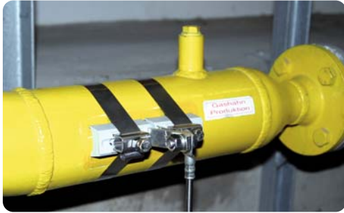
Pipe clamp for safe electrical contacting of pipes in Ex areas for implementation of lightning equipotential bonding according to IEC 62305-3 EN 62305 (VDE 0185-305-3)
